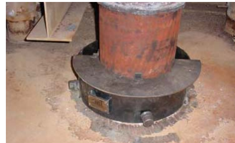
HRSG roof penetration (top cover partially installed)
